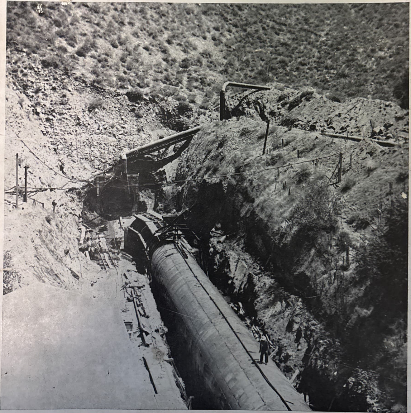
District construction crews close in the last gap in the building of the main line of the Colorado River Aqueduct. Picture shows Casa Loma Siphon at West Portal of San Jacinto Tunnel.
