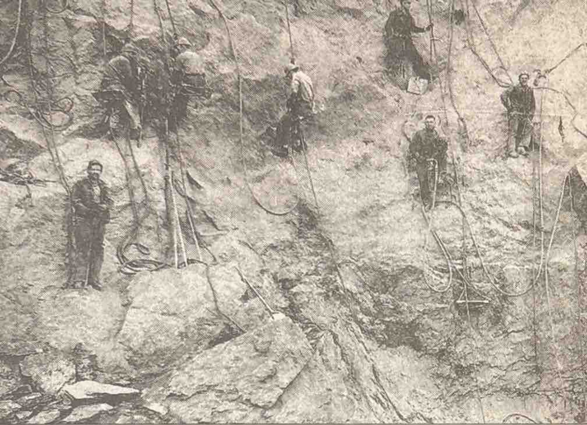
High-scalers pose with their jackhammers during construction of Black Cross is fourth from right.
