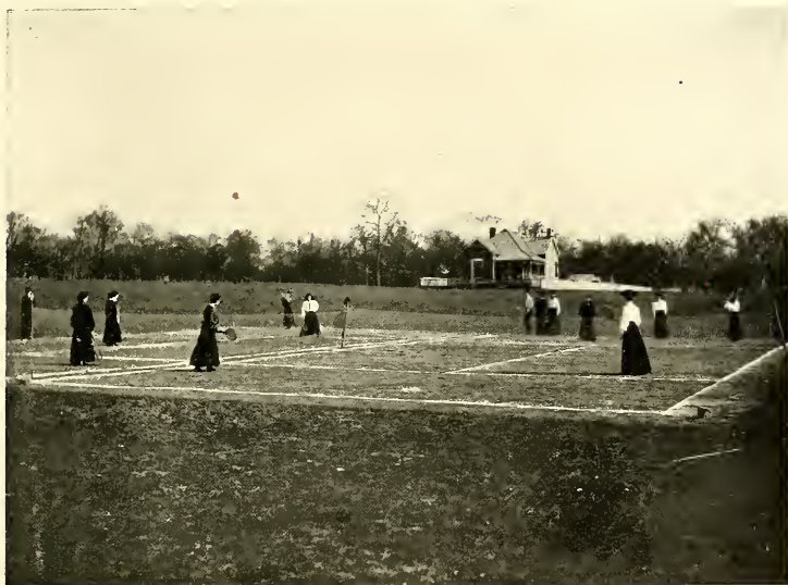
COUNTRY CLUB—TENNIS COURTS II. AND III., CLUBHOUSE
