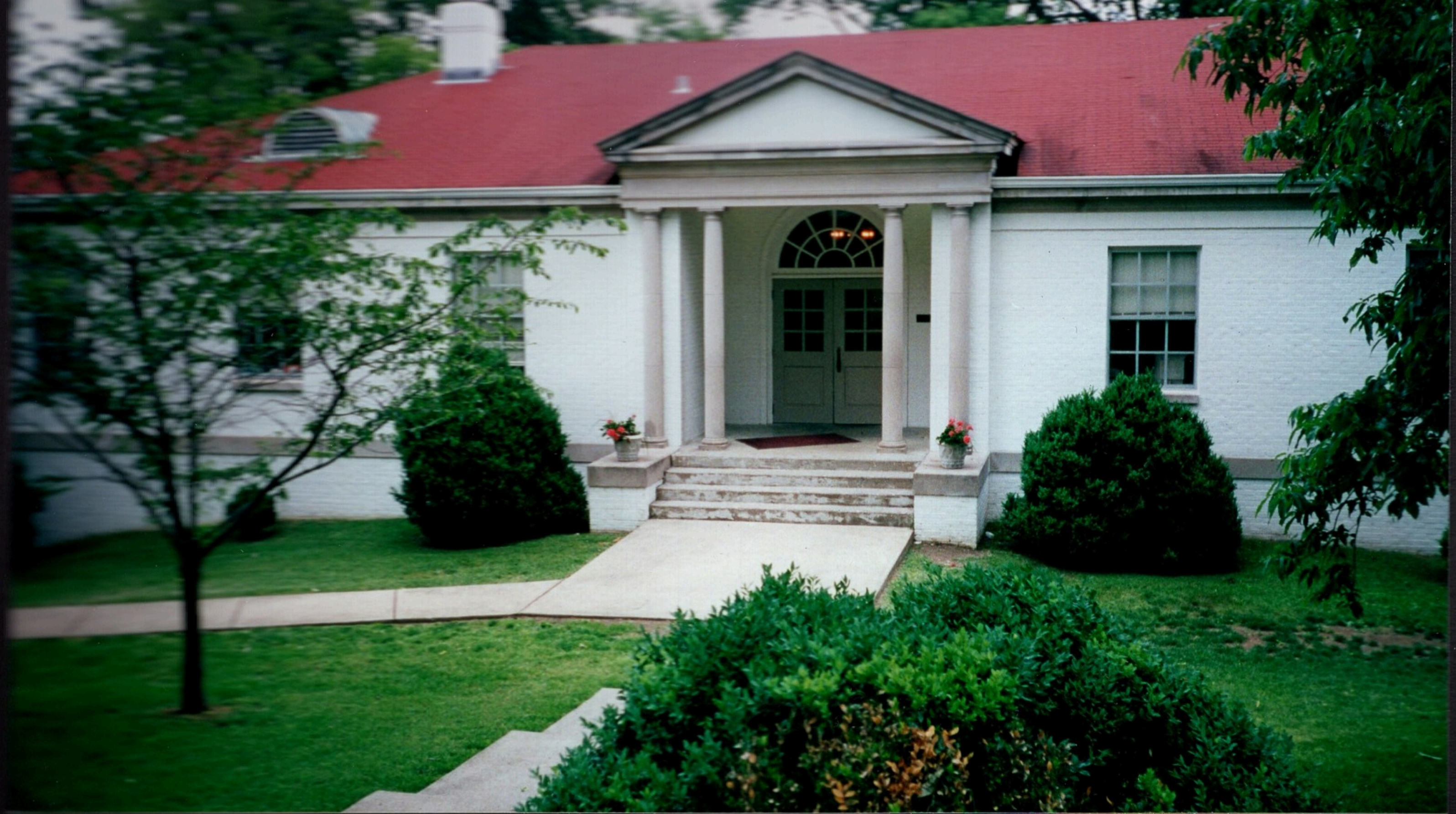
5th & 6th Grade Building
