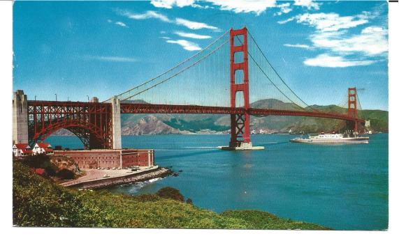
GOLDEN GATE BRIDGE This great suspension bridge, connecting san A Francisco with Marin County in California, has a center span of about four-fifths of a mile and is held some 250 feet above the tides by the works. enormous cables, each made up of more than 8-D 25,000 strands. Mies In Stevens
