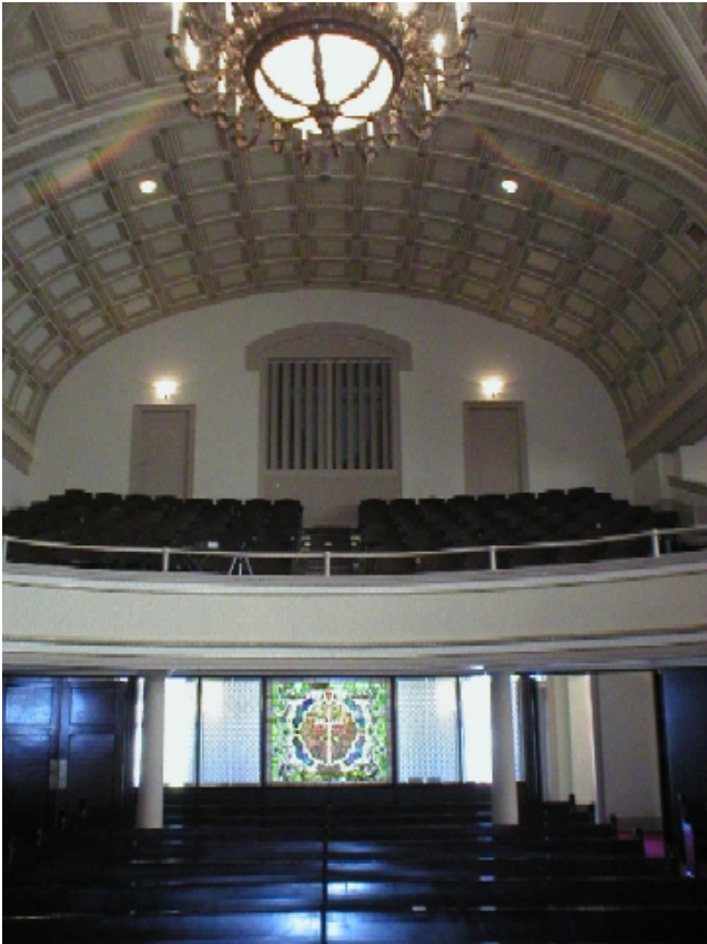
LEFT: The Antiphonal division of the First Christian Church's pipe organ is installed behind the balcony.
