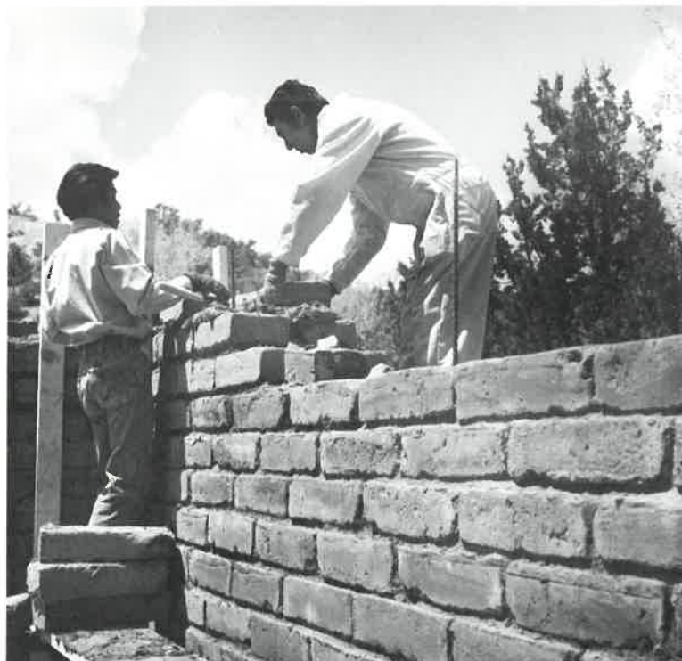
Construction of the Visitor's Center at Nambe Falls. Photo by Mark Nohl.
