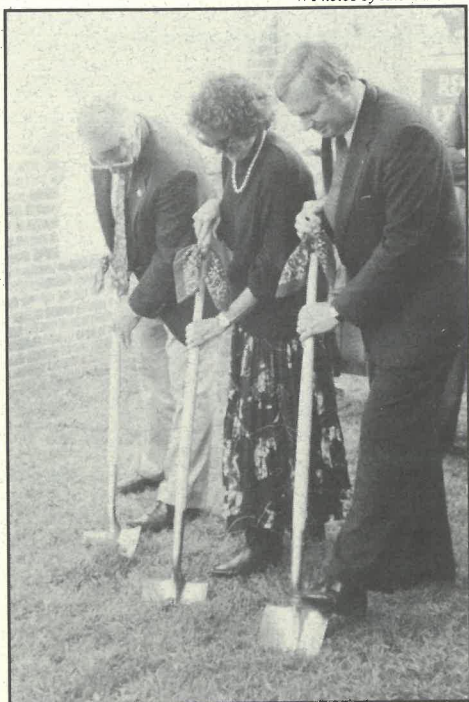
At the climax of the festivities, Dick and Mignon Goetz DeShon and Bill Carpenter broke ground.
