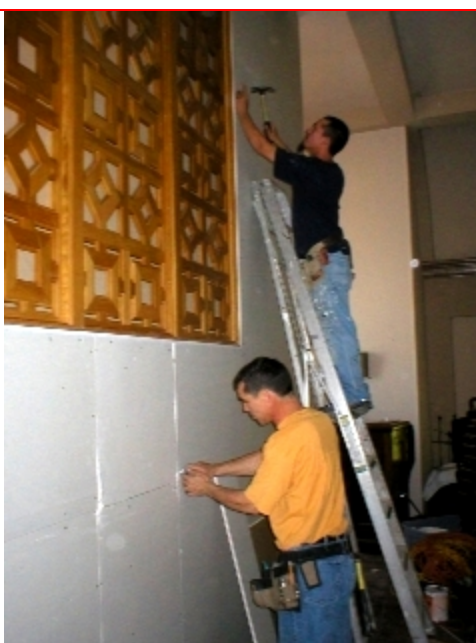
Since the previous organ was self-contained in a cabinet, a room, called an "organ chamber", was constructed in the choir loft by Steve Clayton of Trinity Restoration. In addition to providing safe "housing" for the pipework, expression shades in the tone opening behind the original grillwork provide volume control for the organ.
