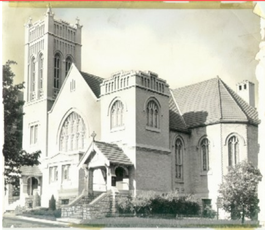
View of the south west corner of building
