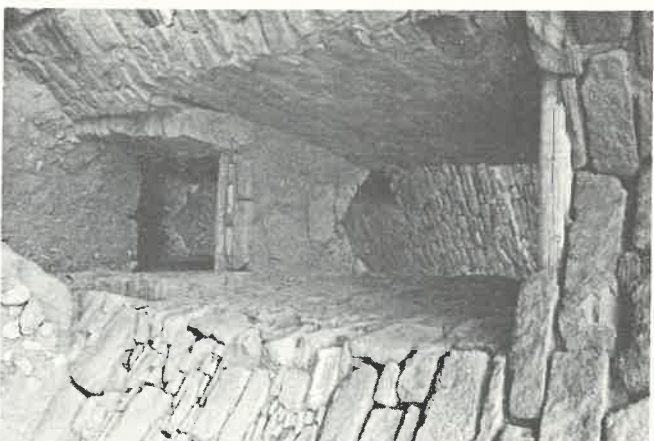
Cross section and photograph of an over-under corner doorway.
