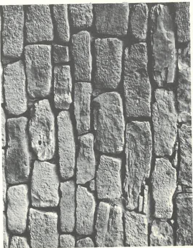
Mesa Verde-style masonry wall.
