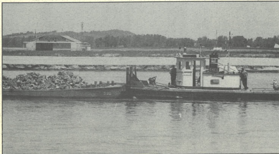
This picture from the archives of the St. Joseph Museum shows the Corps of Engineers working on the Missouri River after the 1952 flood. Rosecrans Airport is in the background.
