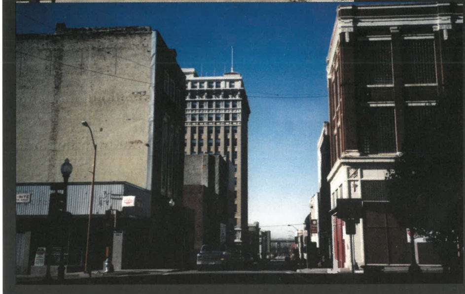
Below: View of Sixth and Felix Streets looking west taken in 1999. Note the extra two floors on the Corby Building. They were added in 1917 to house the St. Joseph Grain Exchange.
