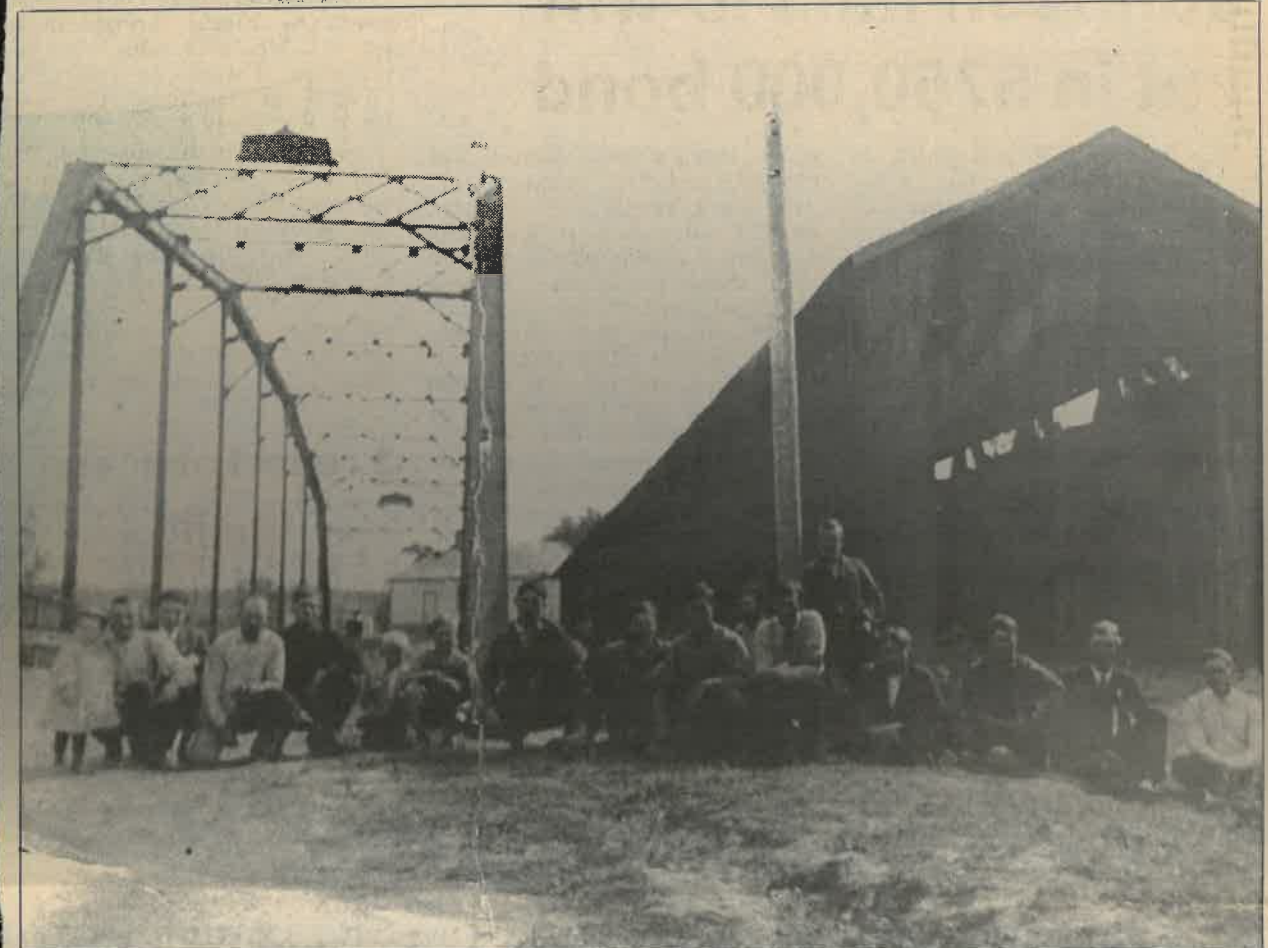
This photo was taken when the old covered bridge near Garrettsburg was to be removed.
