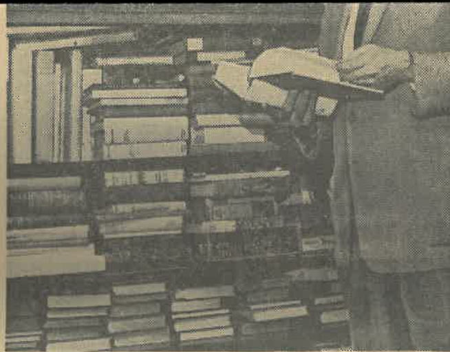
A BOOKCASE DOUBLE STACKED with pamphlets and volumes describing the deeds of heroes and outlaws of the West, is examined by Theodore J. Ismert, the oldest of Ismert's four sons. The collection, estimated in size at more than 10,000 volumes, overflows into several rooms at the Ismert home.
