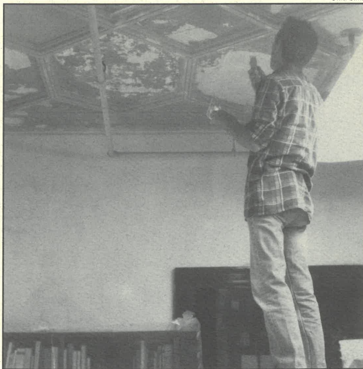
Chris Fisher prepares the library ceiling for painting. A combination of colors will be used to emphasize the architectural features of the room.
