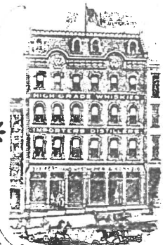
EASTERN OFFICES, 317-319 MAIN ST. CINCINNATI, O.
