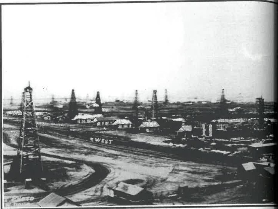
Figure 14. Panoramic view of the oil field town of Midian, Kansas, looking northwest from the top of an oil derrick ca. 1918 (courtesy of the Butler County Historical Society).
