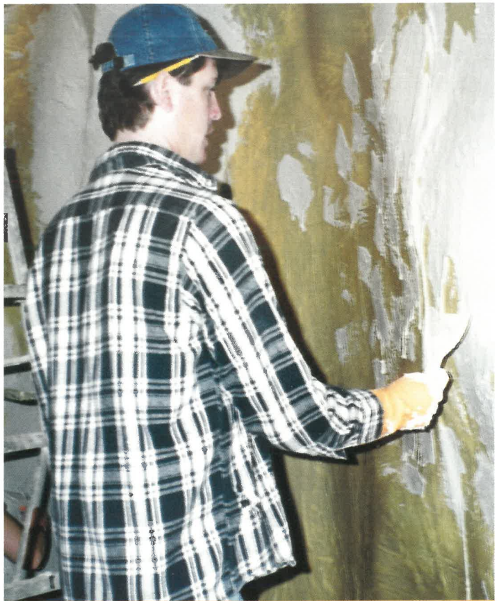
Robbie Sipes plasters the walls of the Gold Rush exhibit. The completed walls will resemble the rock walls of a mine.
