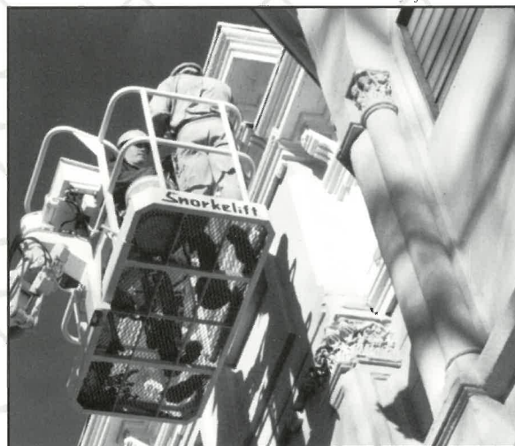
L to R: Robbie Sipes and David Mead place anchors for the strings of lights.
