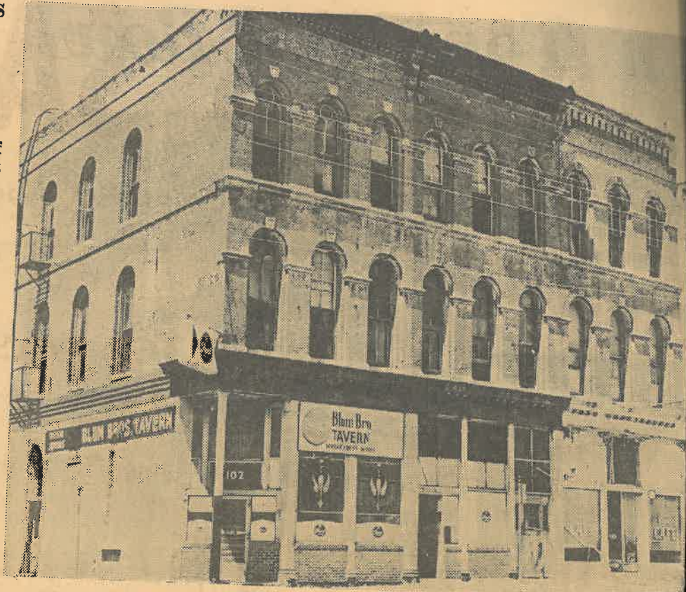
Back in 1900 the Colonial Hotel, 2d and Felix street, which houses Blum Brothers Tavern, was in the heart of the city's business center. Now the building will be razed to make way for one of the new West Belt highway ramps.
