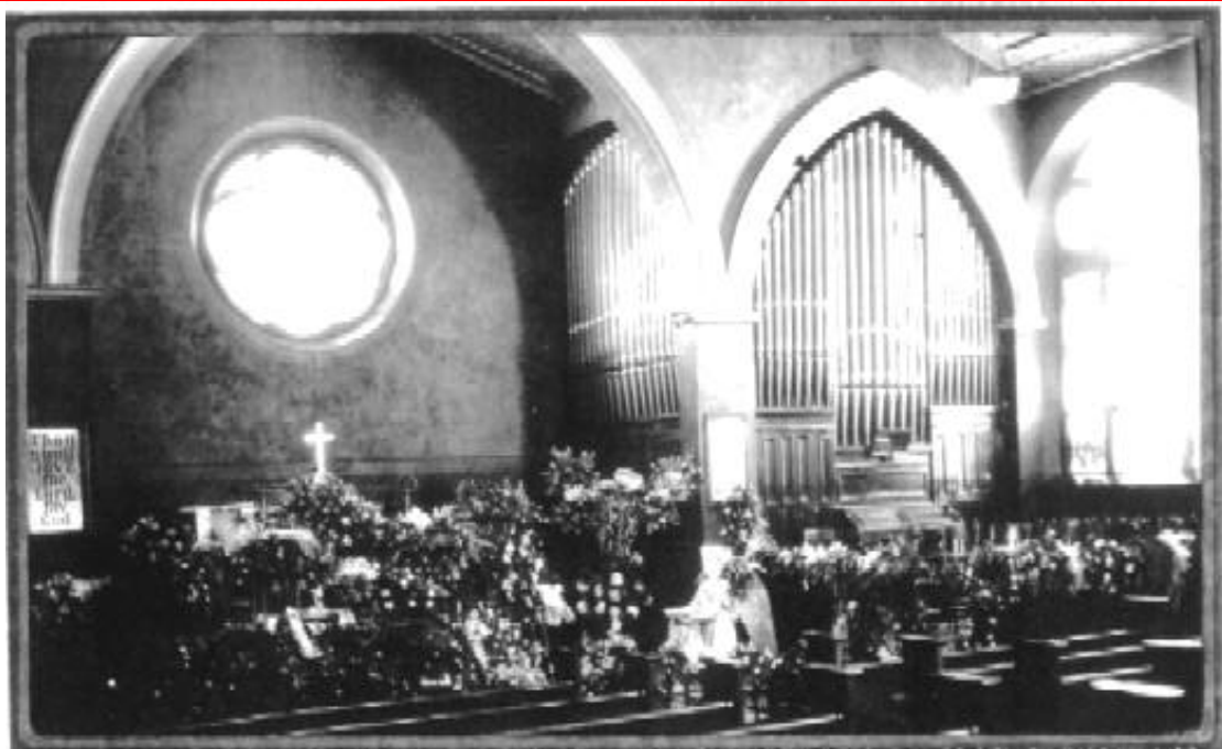
Original Moller organ installation
