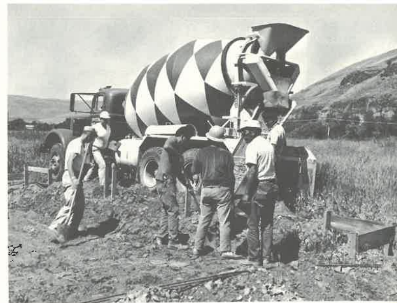
Nez Perce Indians pouring foundations for a development of reservation dwellings to be constructed under the Mutual Help Housing Program. (PHOTO: BUREAU OF INDIAN AFFAIRS)
