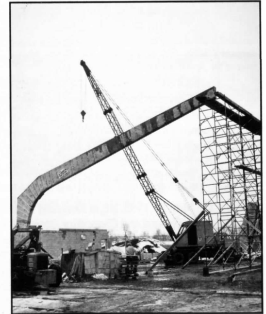
Construction of the New Lenox campus began in May of 1961.
