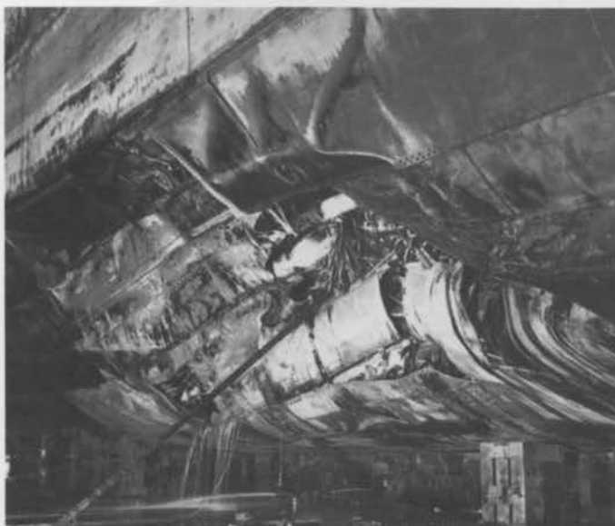
Torpedo damage to CANBERRA , as seen in the floating drydock at Manus, British Admiralties, late 1944.
