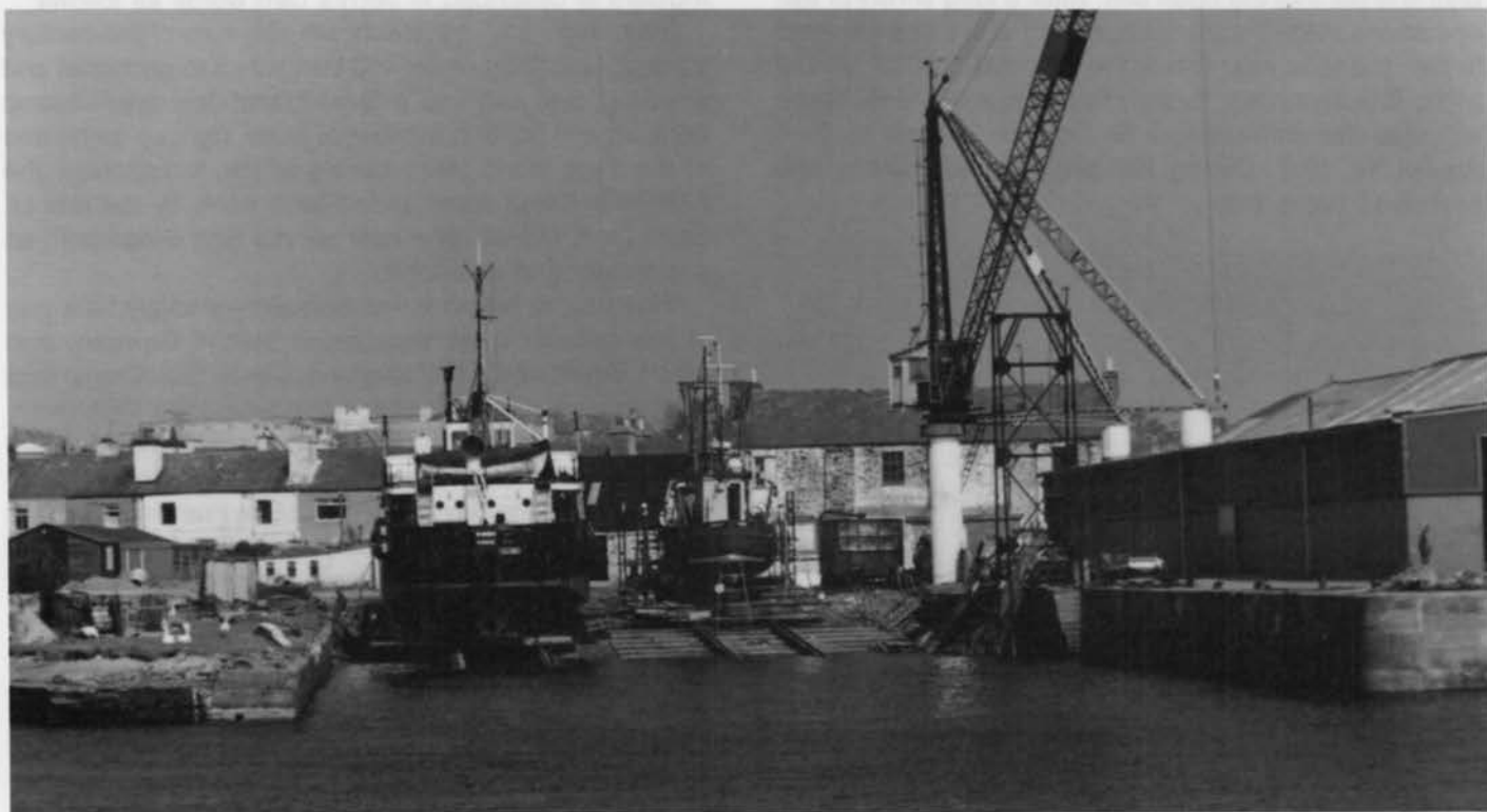
The shipyard where EUTERPE was built, Ramsey, Isle of Man. The EUTERPE went down the ways where the large vessel at left is resting. The stone house in the center background was there when the ship was launched.
