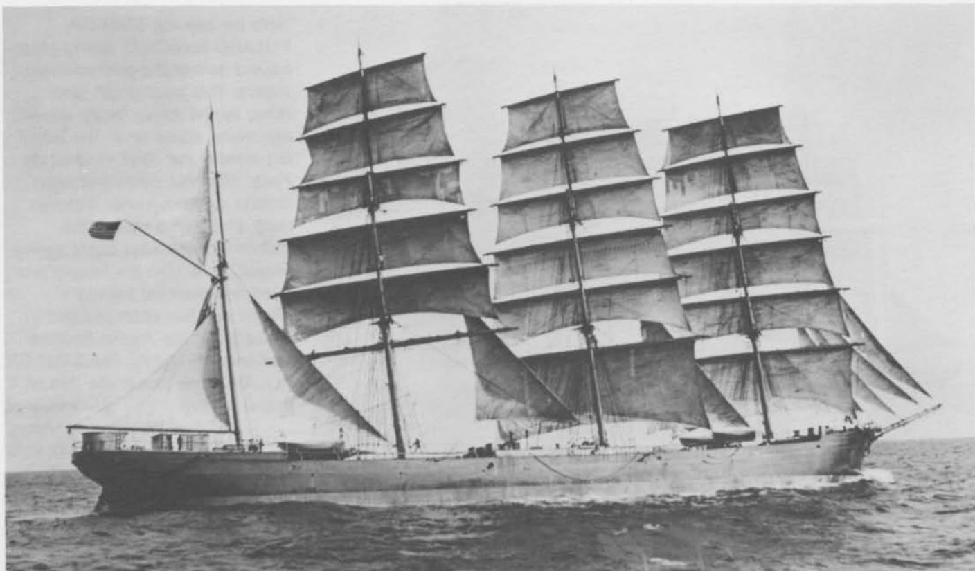
The big four-masted bark STAR OF LAPLAND (ex-ATLAS) sails on a starboard tack in this view. Two men are working on her mizzen course and a gaff tops'l is set on the jigger. Built of steel in 1902, the LAPLAND was one of the newer Packers' ships. She startled her owners in 1917 by sailing from San Francisco to Bristol Bay in seven days, five hours. In 1936 she was sold to the Japanese.
