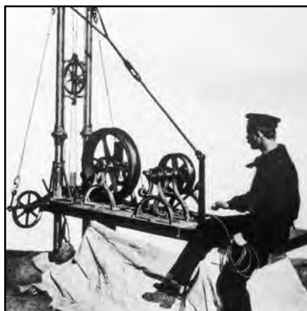
The Sigsbee Sounding Machine rigged for paying out.
