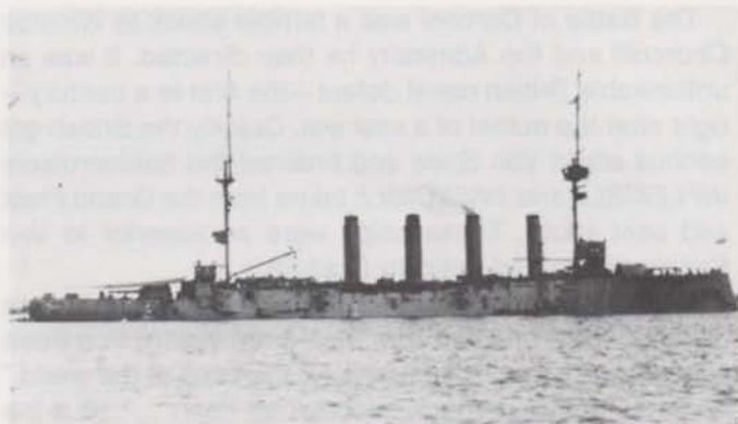
H.M.S. GOOD HOPE, armored cruiser, flagship of Cradock's squadron. Launched in 1901, she carried two 9.2-inch guns and a variety of smaller armament on a displacement of 14,100 tons. Her crew numbered 900.
