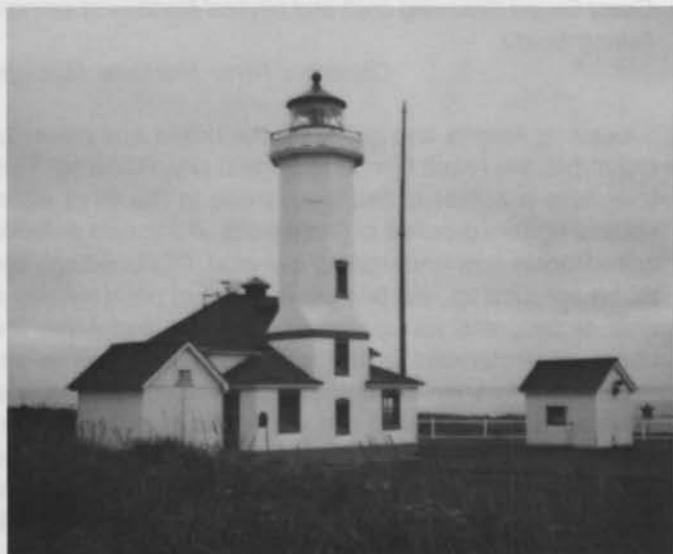
Pt. Wilson Light at the entrance to Puget Sound, just north of Port Townsend.
