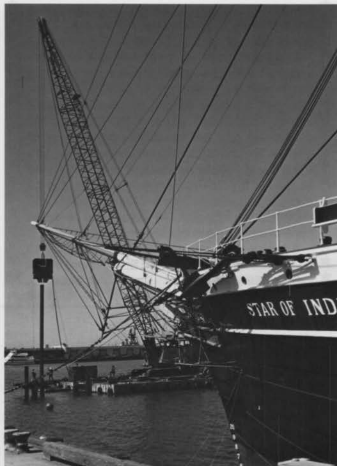
This photo shows an early stage of construction on the Maritime Museum's new pier for BERKELEY and MEDEA . Pilings are driven to provide support for the floating pier.
