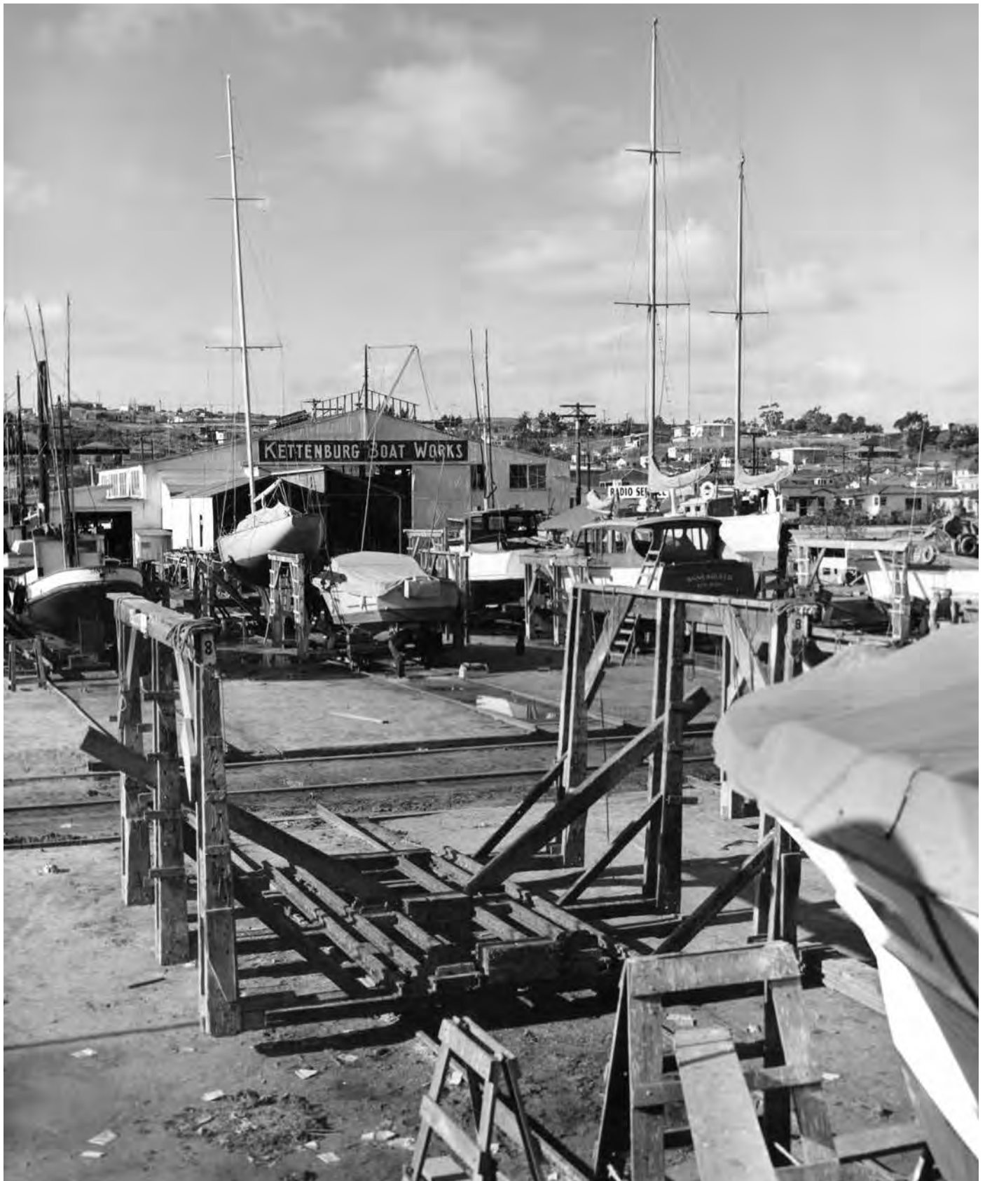
The Kettenburg yard in the early 1950s, looking toward the west. The sailboat on the cradle to the left is Gartz Gould's PCC Ballerina , a very successful racer. The main boat construction building was built of corrugated galvanized iron in 1929.
