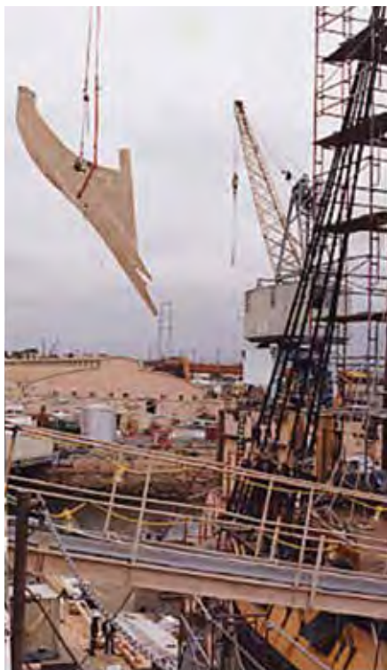
In Spring 2002, the new stem is “flown” into place in San Diego. It fit snugly.
