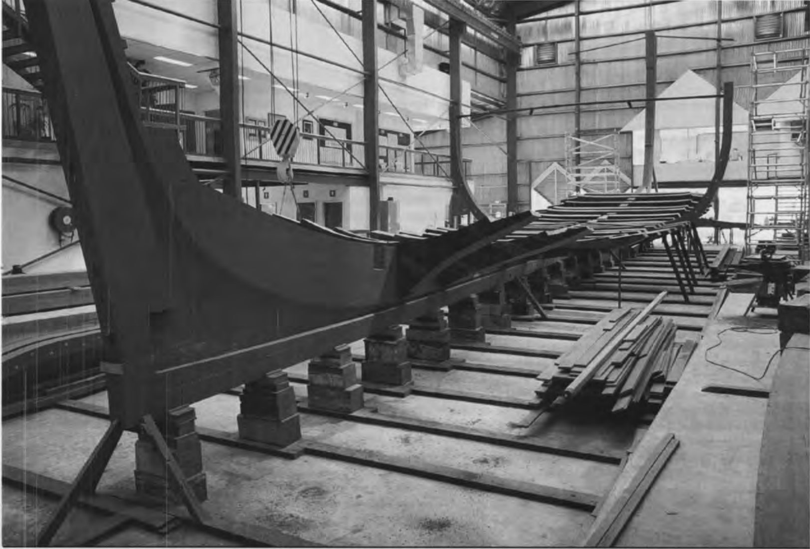
Above: After the ship shed was assembled, the prefabricated keel, stem post, stern, and floors were transported to the shed and set up. (Courtesy HM Bark Endeavour Foundation).
