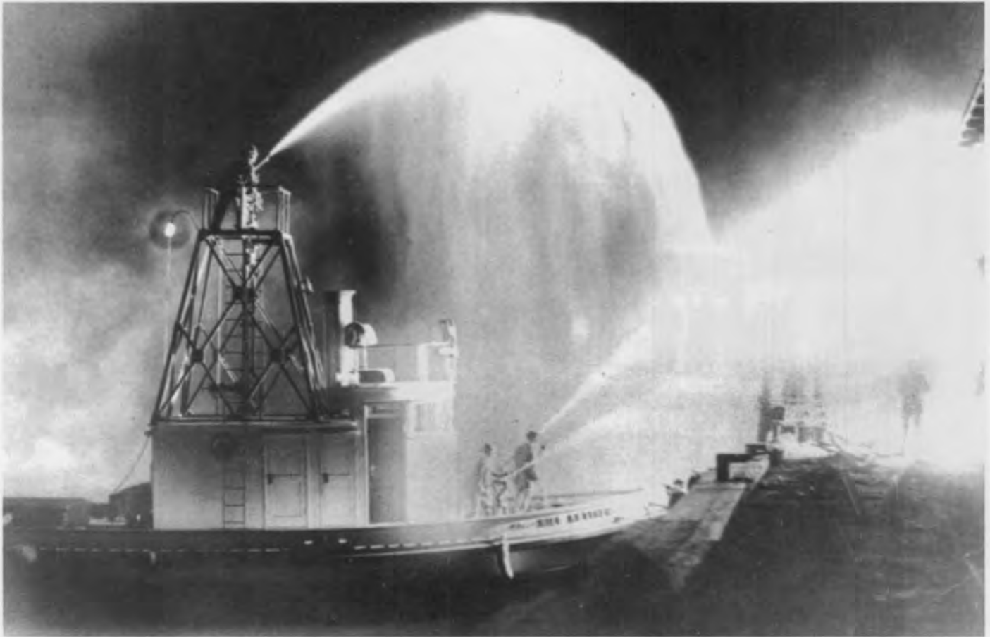
At work on the Star & Crescent Company's boathouse in 1930.
