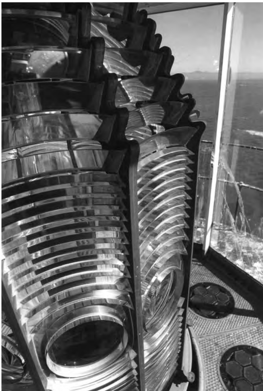
The 1887 third order Fresnel lens stands unused today atop the tower.
