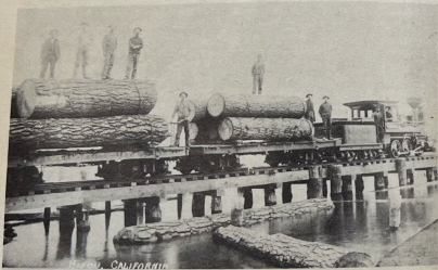
Engine "Santa Cruz" on the pier at Bijou, Calif.
