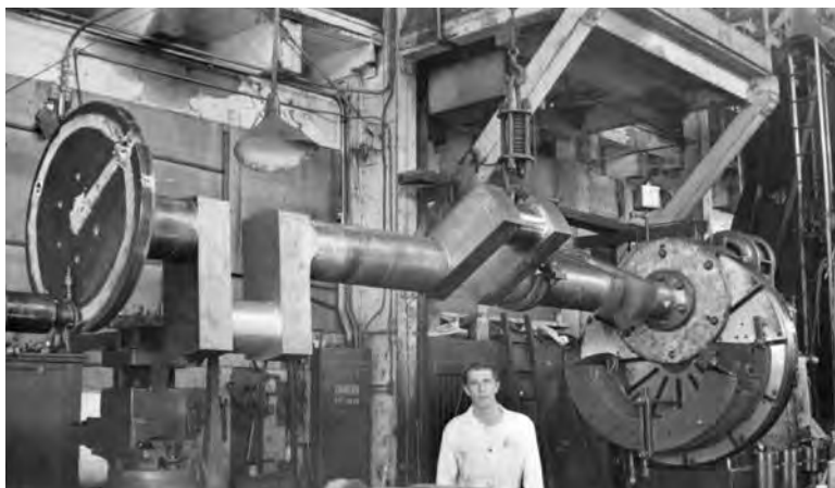
This replacement for Berkeley's huge crankshaft was made at Moore shipyard in San Francisco in the 1950s.
