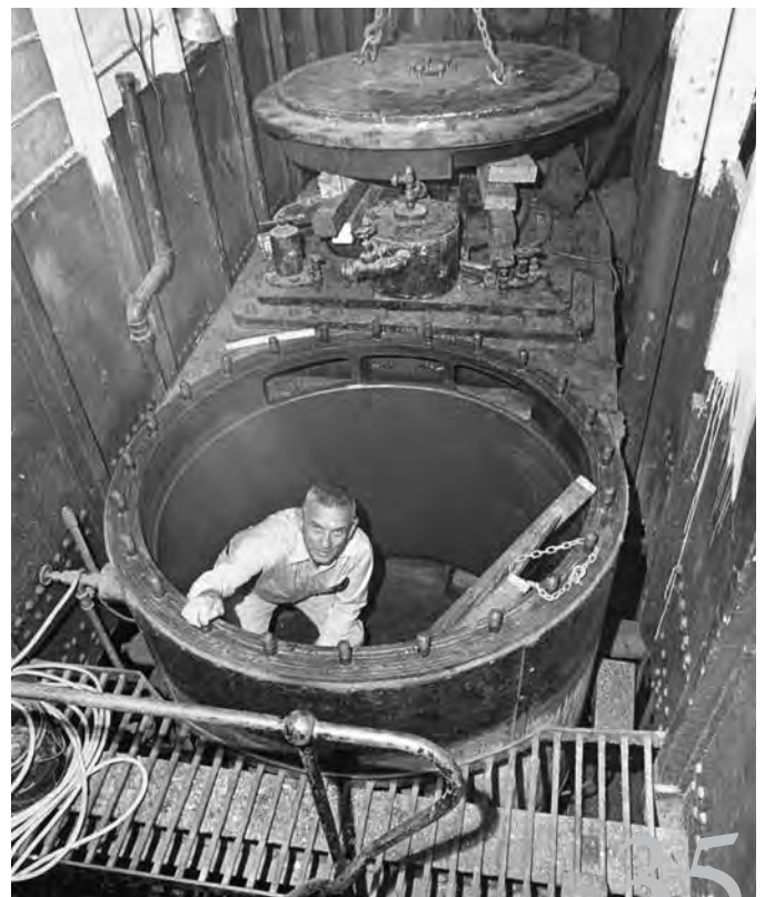
Berkeley's powerplant originally featured Scotch marine boilers like this
