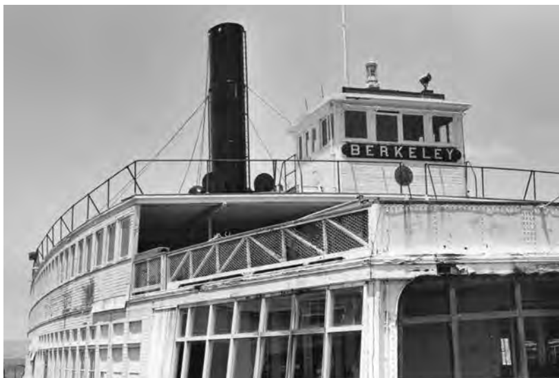
Cracked and peeling paint and exposed rotted wood disfigure Berkeley in 1973. Museum volunteer Winn Bagley wrote that “she could best be described as a basket case. She had lain for fifteen years in total neglect.”
