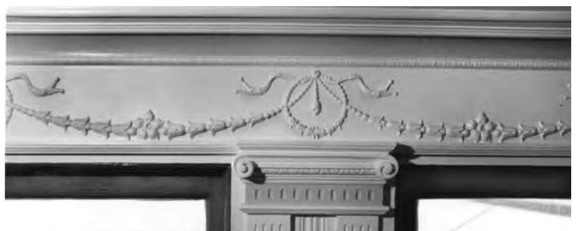
Once the layers of paint at left were stripped away from the ornate frieze on the passenger deck, the fine details of the original emerged again.
