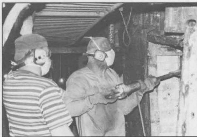
Much work has been done in recent months to restore the BERKELEY's boiler room. Working conditions were difficult in this dim, dirty, and cramped environment. These are Museum employees Bob Crawford (left) and Jim Davis (right) wearing the protective gear needed for this job.
