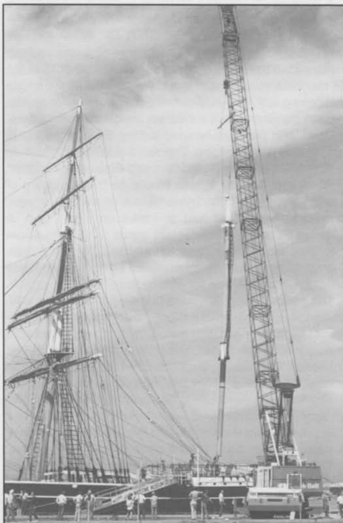
The STAR OF INDIA's mizzenmast is hoisted out by crane for repairs.
