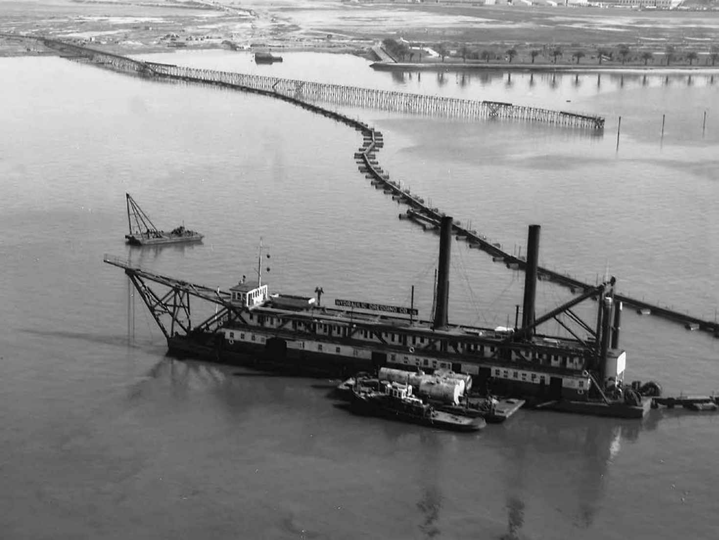
Dredging underway in April, 1939.
