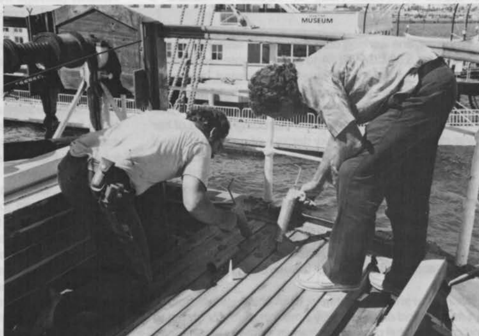
Here crewmen put the caulking in the rabbets. Note wheelbox removed at left, to lay planks underneath.
