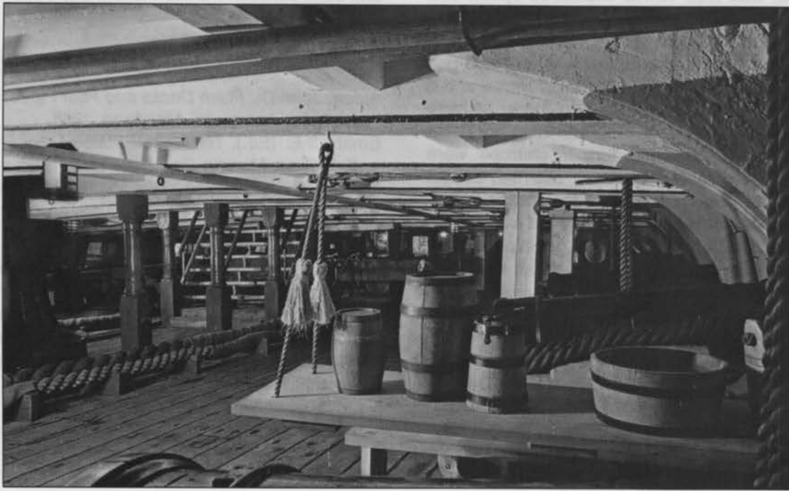
HMS VICTORY's lower gun deck, housing her main battery at 12-foot intervals. The table in foreground was lashed up to the overhead prior to going into action.
