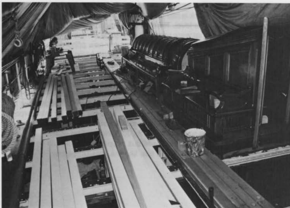
Some of the new planks are fastened down while others are ready.
