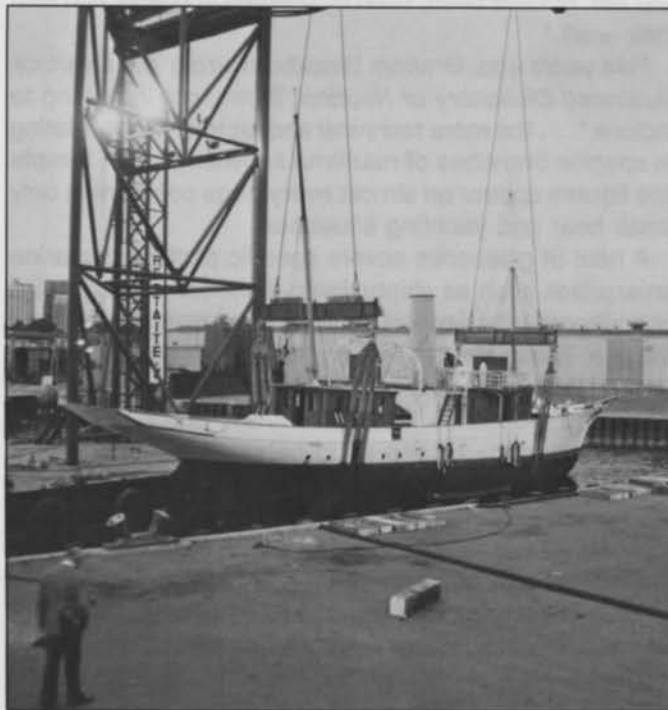
MEDEA is lifted by floating crane onto the dock at 10th Avenue Marine Terminal, San Diego, for her revolutionary hull repair job.
