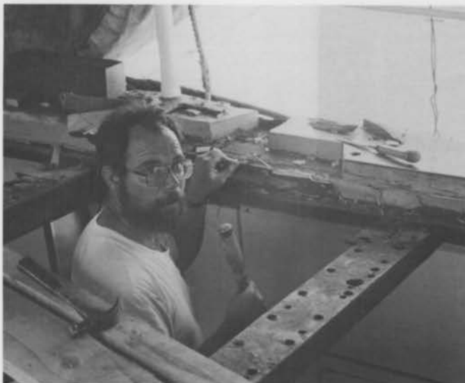
No, this is not a seagoing gnome popping forth from its cave—but our very own carpenter, Jeff Saar, as he puts in many hours on the deck job.
