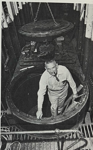
No, Junior, this is not a gnome emerging from a cave; it is our hard-working Port Engineer, Ed Paxton, climbing out of the low-pressure cylinder of the Berkeley's main engine. Behind him, suspended by two chains, is the massive cylinder-cover. (Photo by Roscoe Smith)
