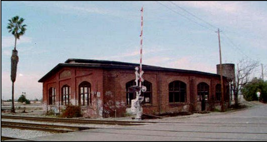
Lenzen Avenue Roundhouse before it was dismantled.
