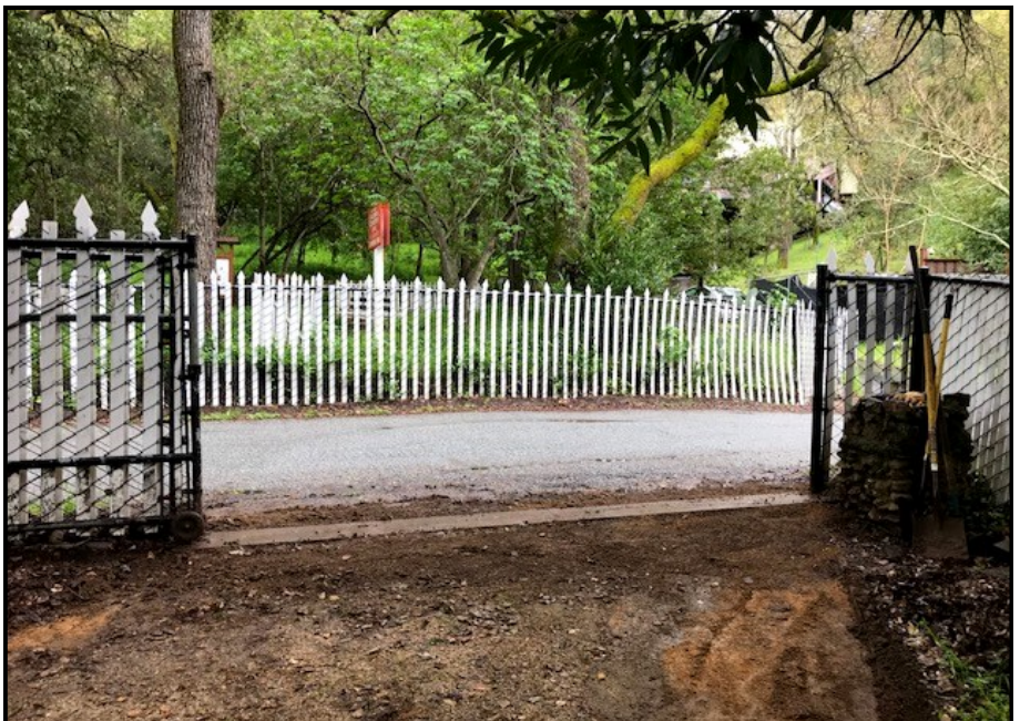
Repaired gate at Hacienda Cemetery. Work done by Eric Johns.
