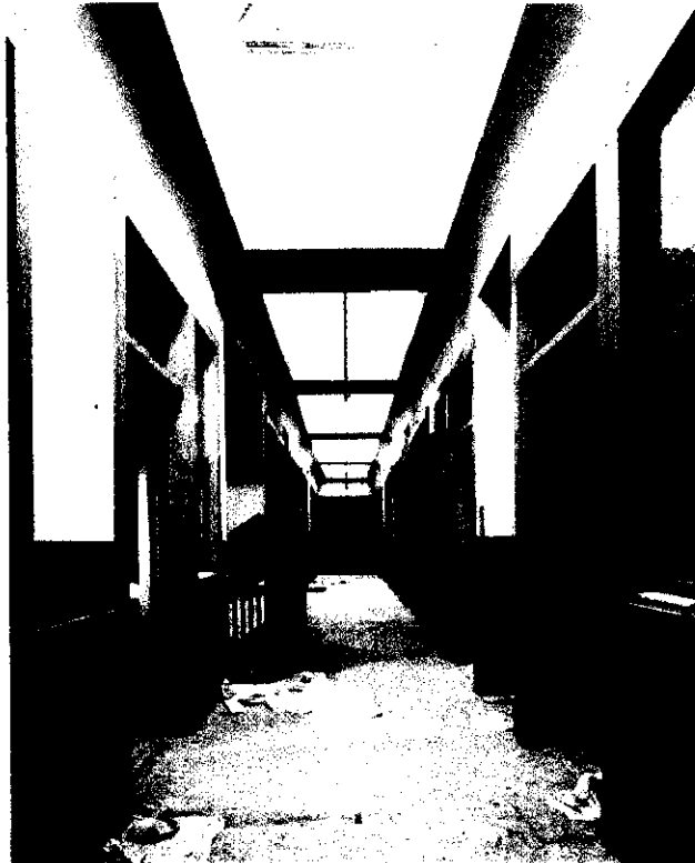
Photograph 5—Second floor hallway before restoration
