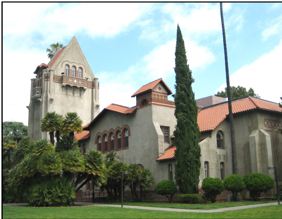
SJSU Tower Hall and Dwight Bentel Hall completed in 1910.
