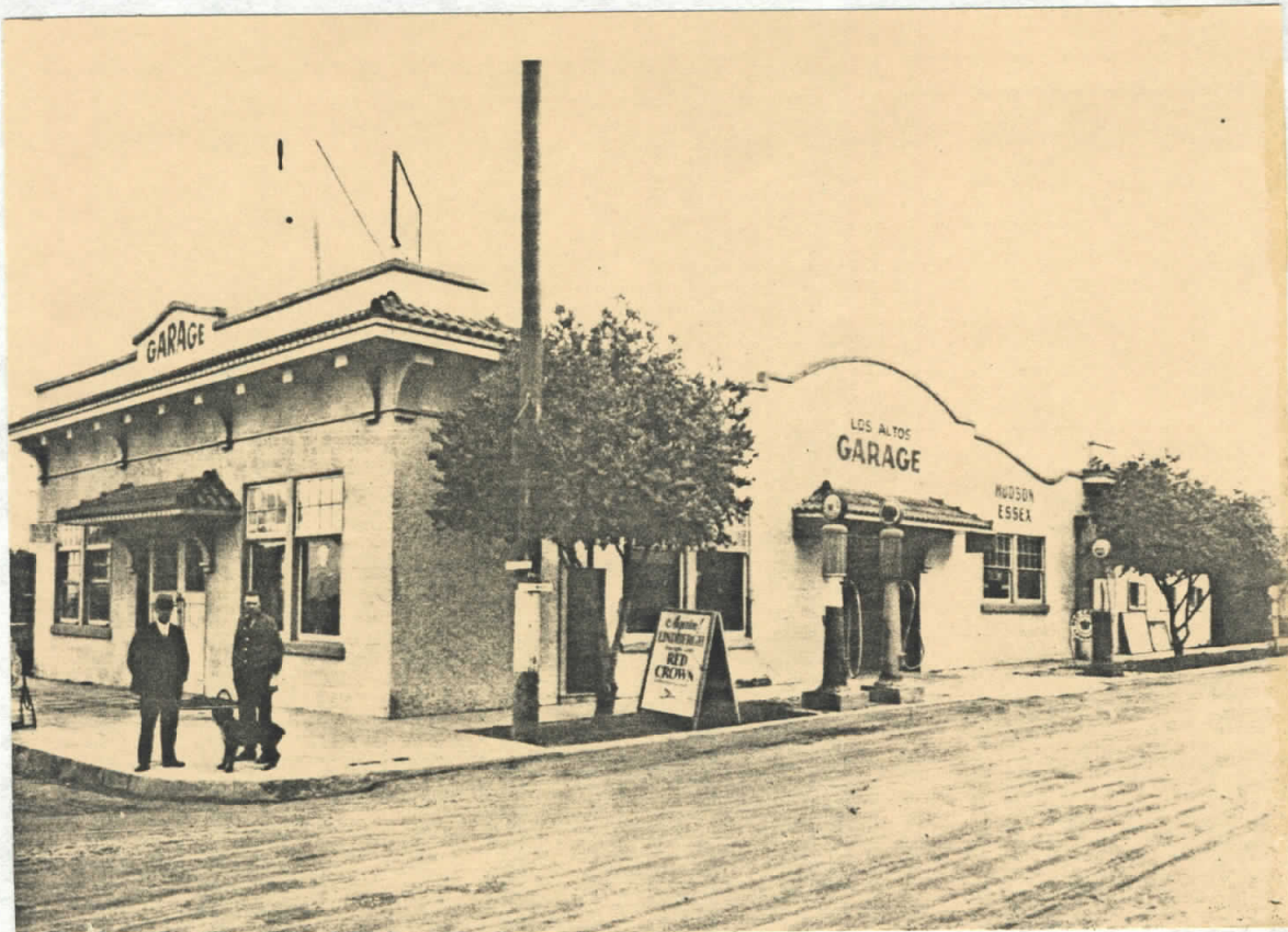
Los Altos Garage-Located on the corner of State St. and 1st. 22.
