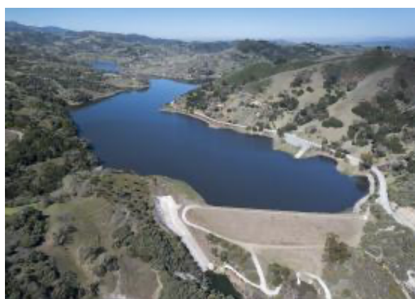
Elmer J. Chesbro Dam and Reservoir (photo: ValleyWater.org)
