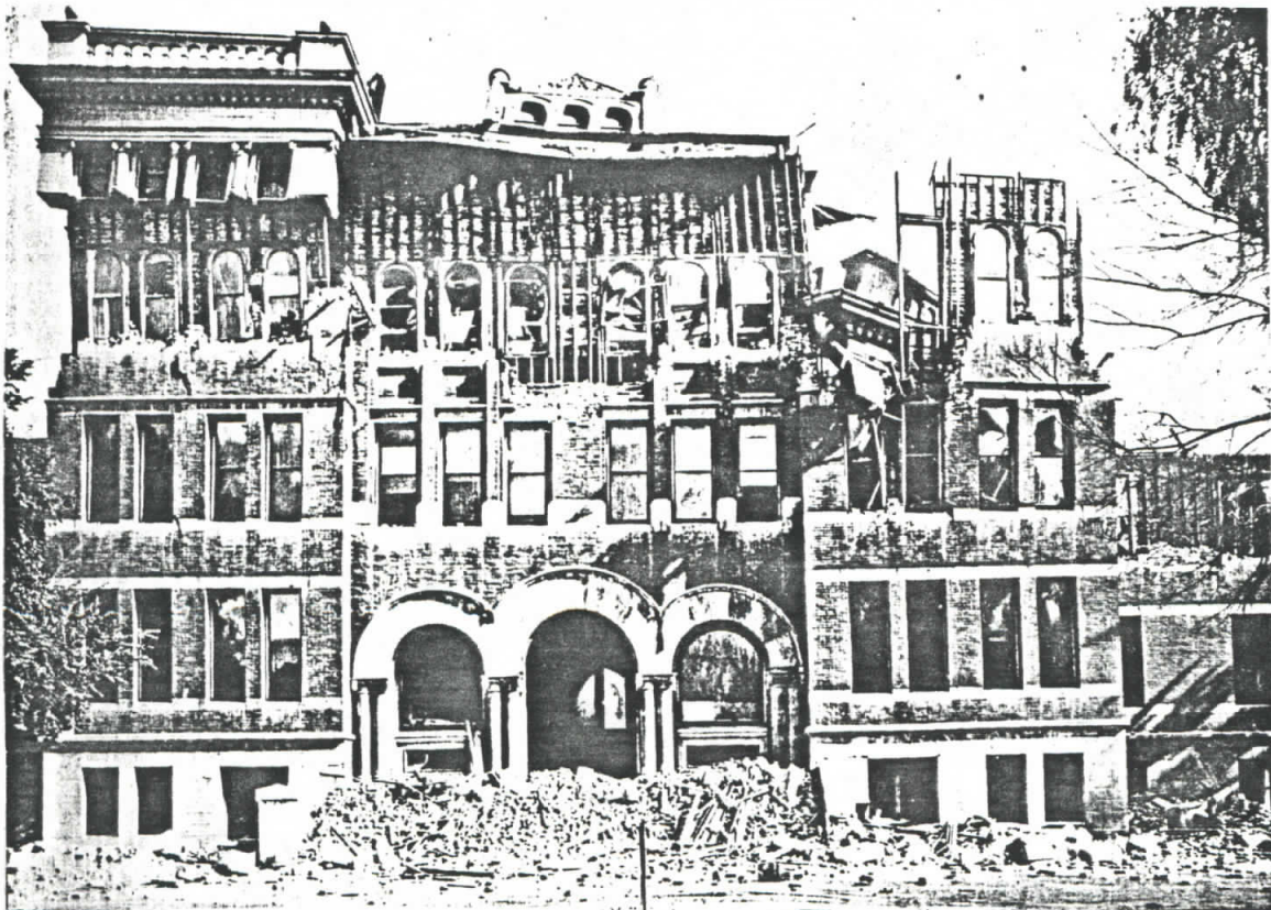
AFTER THE EARTHQUAKE OF 1906
