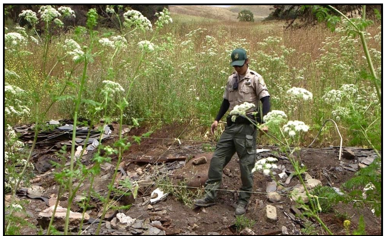
Below right, a year after the fire, spring 2018, vegetation has grown back and an excavation grid has been set up. Debris on the ground includes slate roof tiles. (Photos: Joe Rosato, Jr.)
