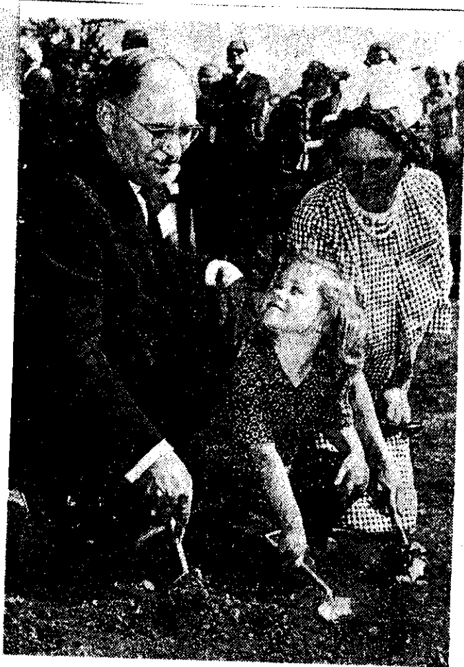
HOSPITAL START — Officials of Good Samaritan Hospital held a sort of Lilliputian ground-breaking at the S. Bascom and National avenue site yesterday. The end result will be anything but small, however, when the $6,500,000, 225-bed structure is finished. Wielding miniature shovels are (left to right) Floyd Sorensen, hospital administrator, Marianne Smith, daughter of a hospital auxiliary member, and Mrs. Gilbert Andrews of Sunnyvale, president of the auxiliary. Construction began immediately.
