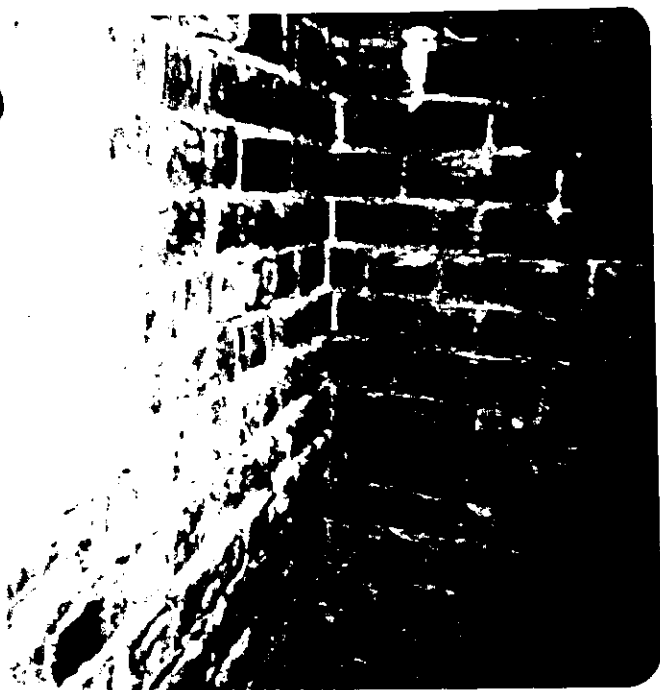
This corner view of the basement shows the all brick foundation.
