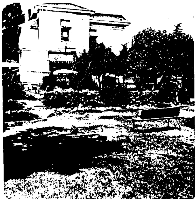
Back view of the house (the original south side). Beyond the awning, upper left, can be seen the filled in porch section.
