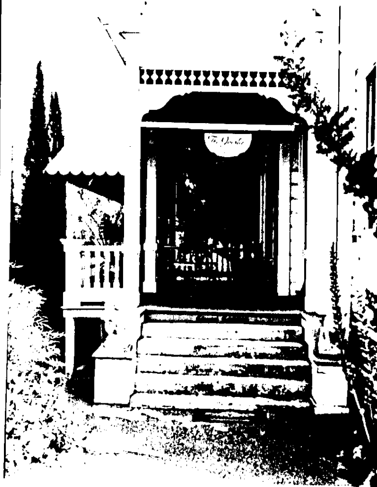
A closer view of the porch shows its size, and some of its architectural importance to the house. Notice the mill work, the wooden awning, the balustrade. A similar balustrade rims the flat roof of the porch. This roof area served two bedrooms as a cool retreat for sleep on warm summer nights.
