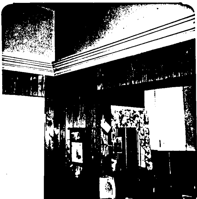
Two walls of the kitchen eating area have this deep, plate rack type molding.
