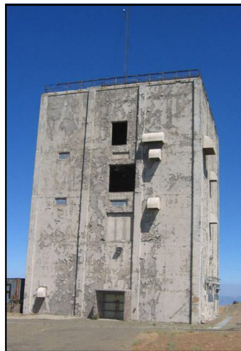
Radar tower, close up view
