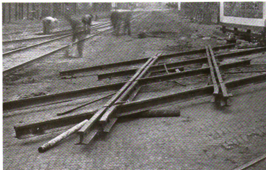
Fig. 5—Acute angle Thermit welded crossing for double track street railway and single track steam railroad intersection.
