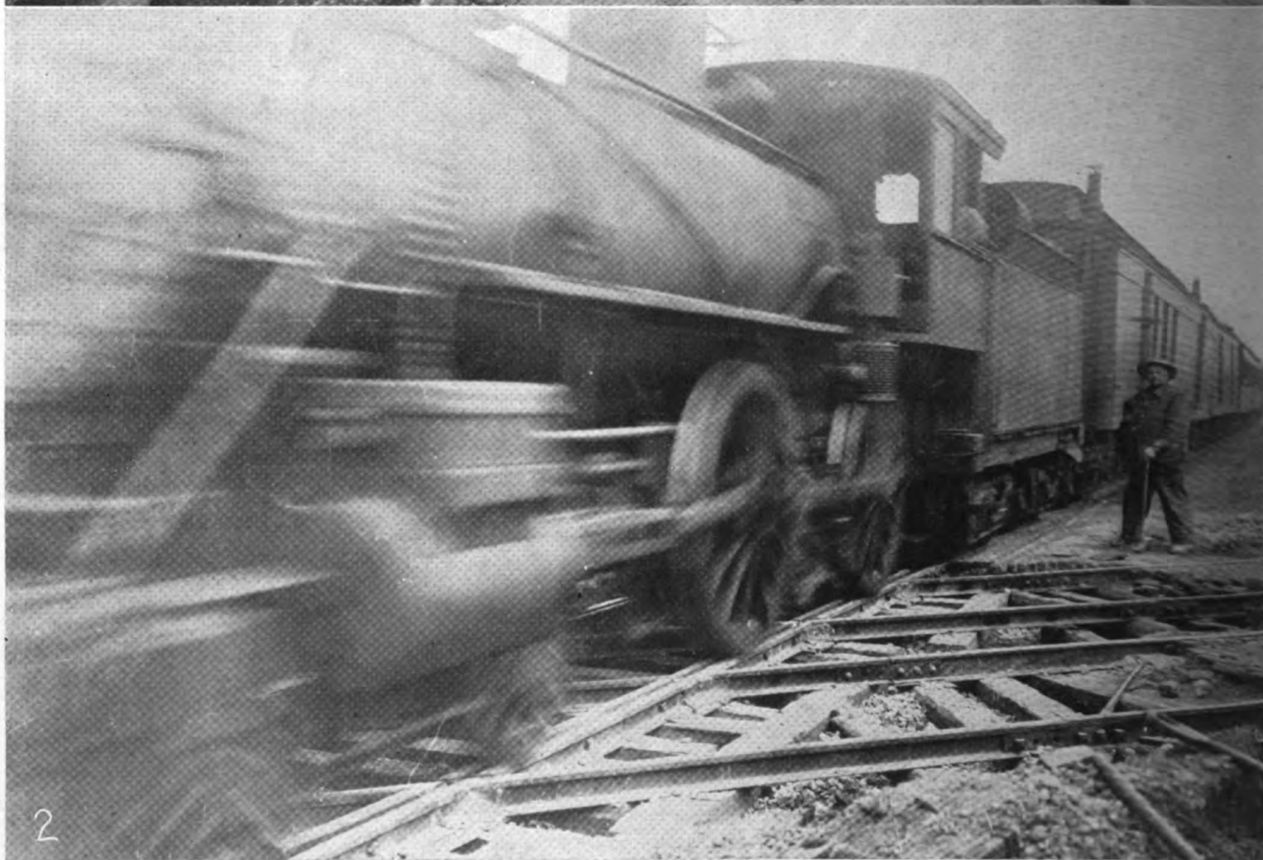
Above—1—Figure 8—Square frog-welded crossing with 100-lb. running rails and 6-inch guard rails. Below—2—Figure 6—Bur-lington railroad train passing over square frog-welded crossing.
