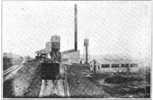
View of Plant Looking North. Main Line of Des Moines & Kansas City on Left. In Order to Make This a Gravity Mine Considerable Filling Was Required with a Pump on the North End of the Yard. Machine Shop and Timber Yard on Right.
