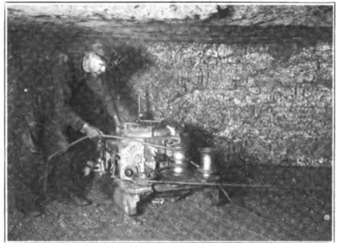
Morgan-Gardner Short Wall Machine Finishing Undercut of Room. Machine Rooms Are 60 Feet Wide, and Undercut 5 Feet Deep and 4\frac{1}{2} Inches in Height Is Made in Less Than One Hour. To Perform the Same Work by Hand Would Require Two Men at Least Six Hours.
