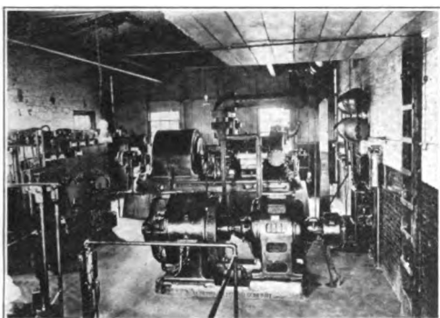
Interior of Engine Room Showing Switch-board on Left, General Electric-Curtis Turbo Driven Generator, 600 K. W., 2,300 Volts, A. C. Current, in the Background, and 100 K. W. Motor Generator Furnishing 250 D. C. Current in Foreground. The Back of This Engine Room Is of Corrugated Iron to Permit Extension for Future Additions.
