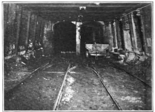
Shaft Bottom Looking West. Concrete Arches Are at Bottom of Shaft. Note Steel Columns and "I" Beams Supporting Sides and Roof.
